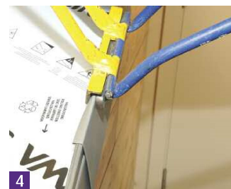
4 Crimp the standing seam at the verge.
