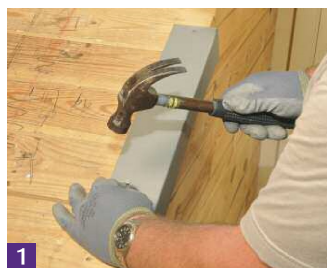
1 Install a zinc clip with nails leaving a 20mm space with the verge.
