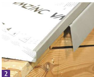
2 Position the standing seam panel.
