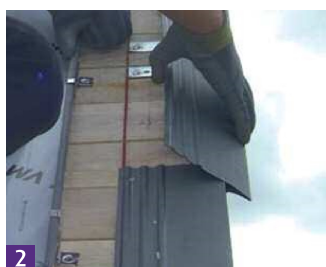
2 Fit the verge strip into the stiffener and fix with nails. The strips should overlap by 50mm.
