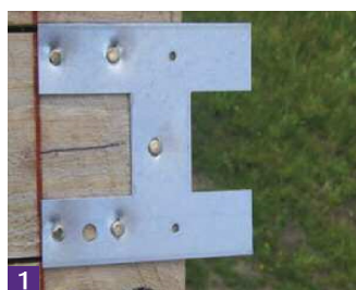
1 Fix the stiffeners at 300mm centres.
