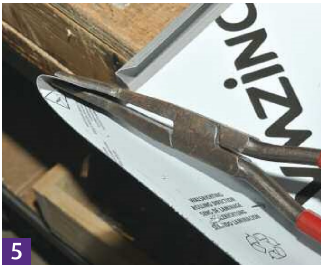
5 Create fold on panel upstand.
