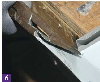
6 Finish fold on panel upstand.
