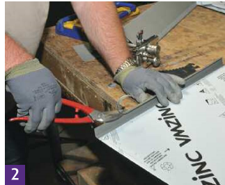
2 Cut away return fold on the profiles.
