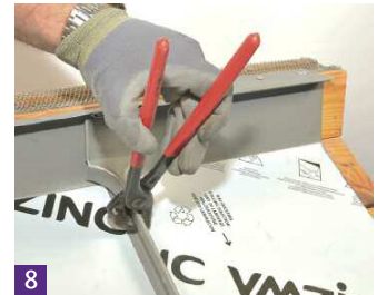
8 Fit saddle piece and pinch at seam.
