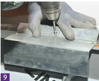
9 Fit clip for ridge flashing.
