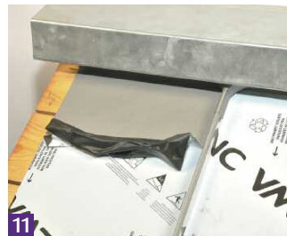
11 Do not partially remove film.
