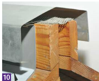
10 Insert ridge flashing.
