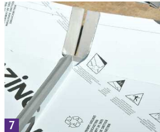
7 Seam panels together.
