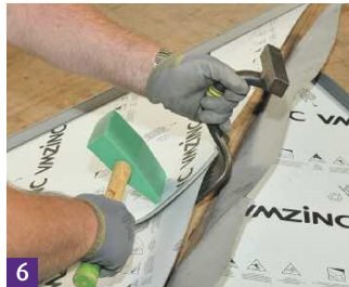
6 The seams are again flattened.
