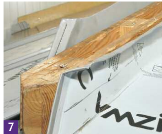
7 The hip batten is installed.
