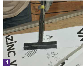
4 The panel is folded upwards.
