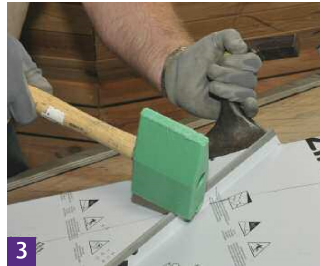
3 The seams are carefully flattened over 150mm.
