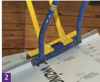
2 The seams are crimped beyond the hip.
