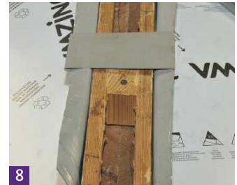
8 A zinc clip is installed prior to the hip flashing being fitted.
