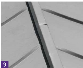
9 The completed hip
