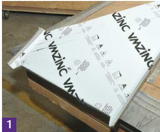
1 Panels are installed on the hip.
