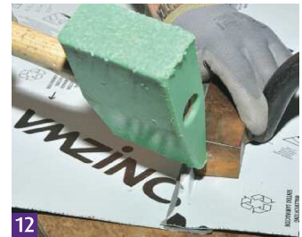
12 Hammer over swept end.
