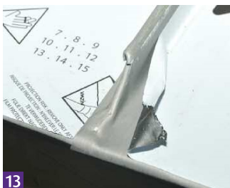
13 Completed eaves prior to film removal.
