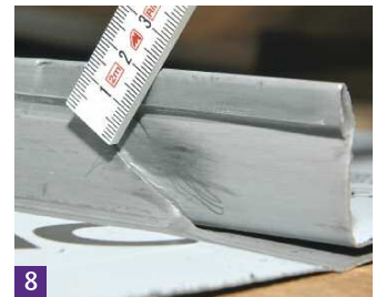
8 Mark the zinc at 15mm above the cut edge.
