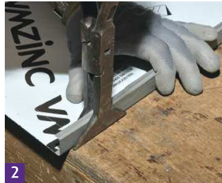
2 Straighten the upstand.
