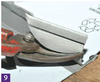
9 Cut the zinc back.
