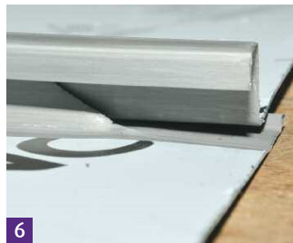
6 Install 2nd panel.
