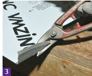
3 Cut back the zinc.
